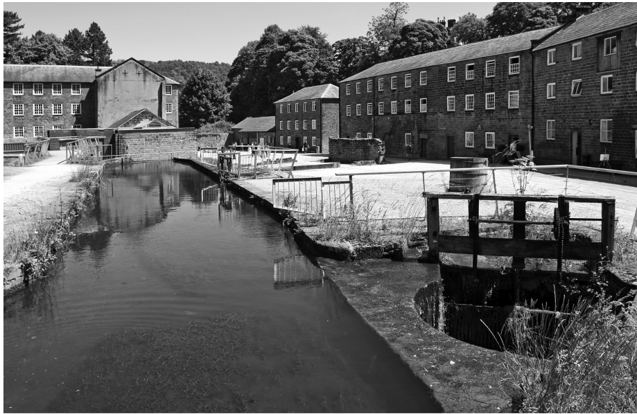
Figure 2.8: Cromford Mill in Derbyshire (UK), where Richard Arkwright built his revolutionary water-powered cotton-spinning frame. Built in 1771-1782, the five-storey mill employed over 200 workers. How useful is the photograph for explaining why Arkwright chose this location for his mill?
